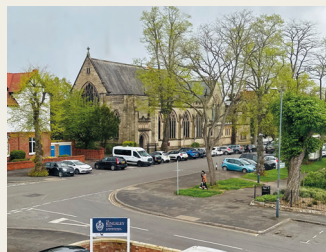
View overlooking Holy Trinity Church taken from a side window Anna Gardner, TKS 1995-2000
